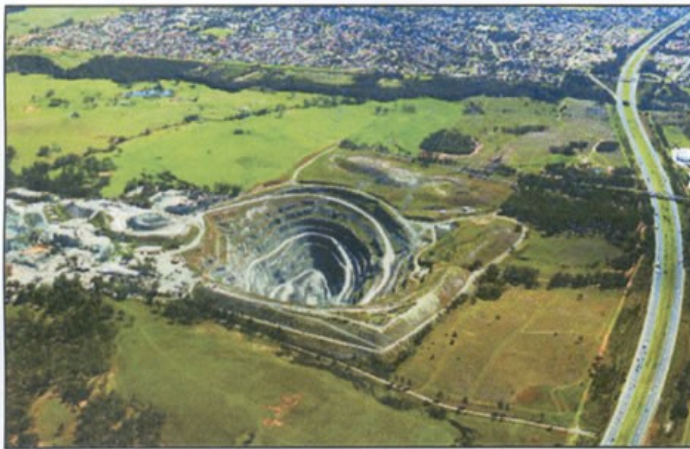
Dial A Dump plans to turn a Sydney quarry into a major dry waste landfill.
